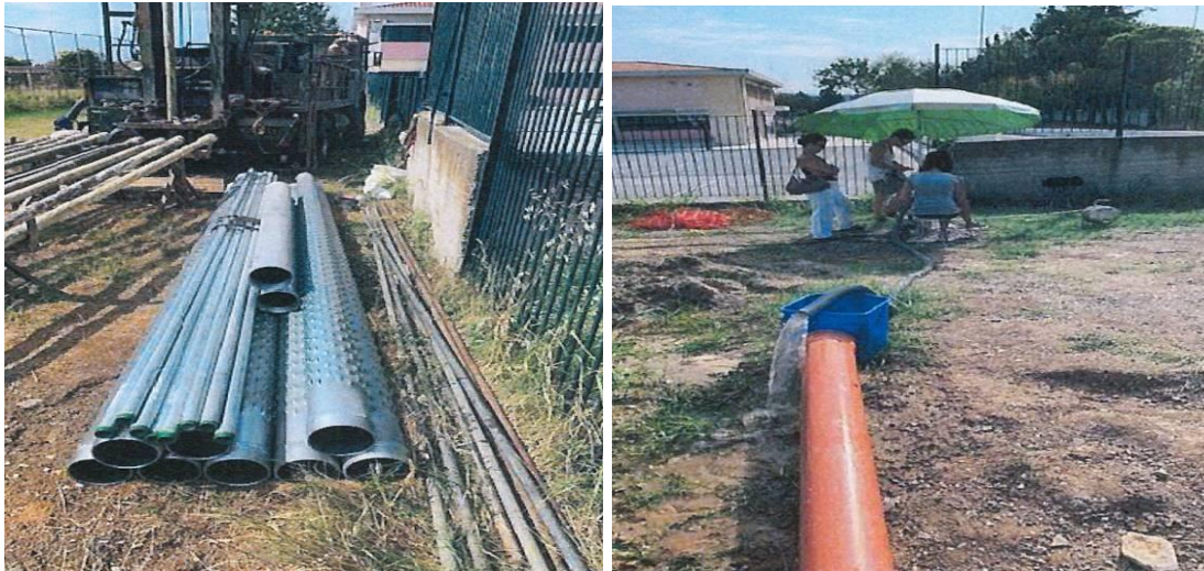
Image 3.1 Photos during construction
