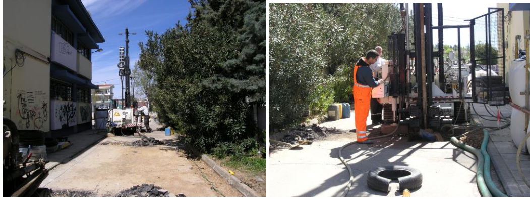
Figure 3. Shallow geothermal drilling (1 st Gymnasium of Pileia)
