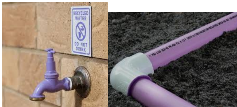
Figure 5.3. Gray water network labeling
