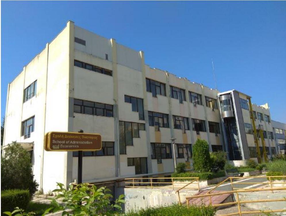
Figure 18. Front and north side view of selected Building B for the studies.
