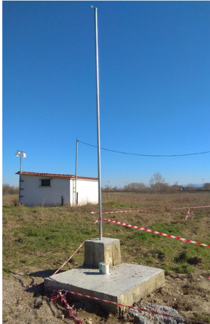
Figure 44. A 6m steel pipe is anchored to the concrete base
