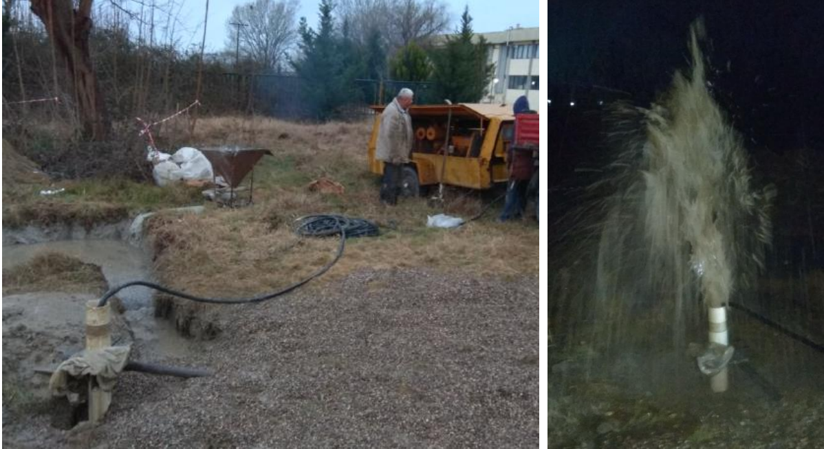
Figure 39. Development of the well using the air-lift technique
