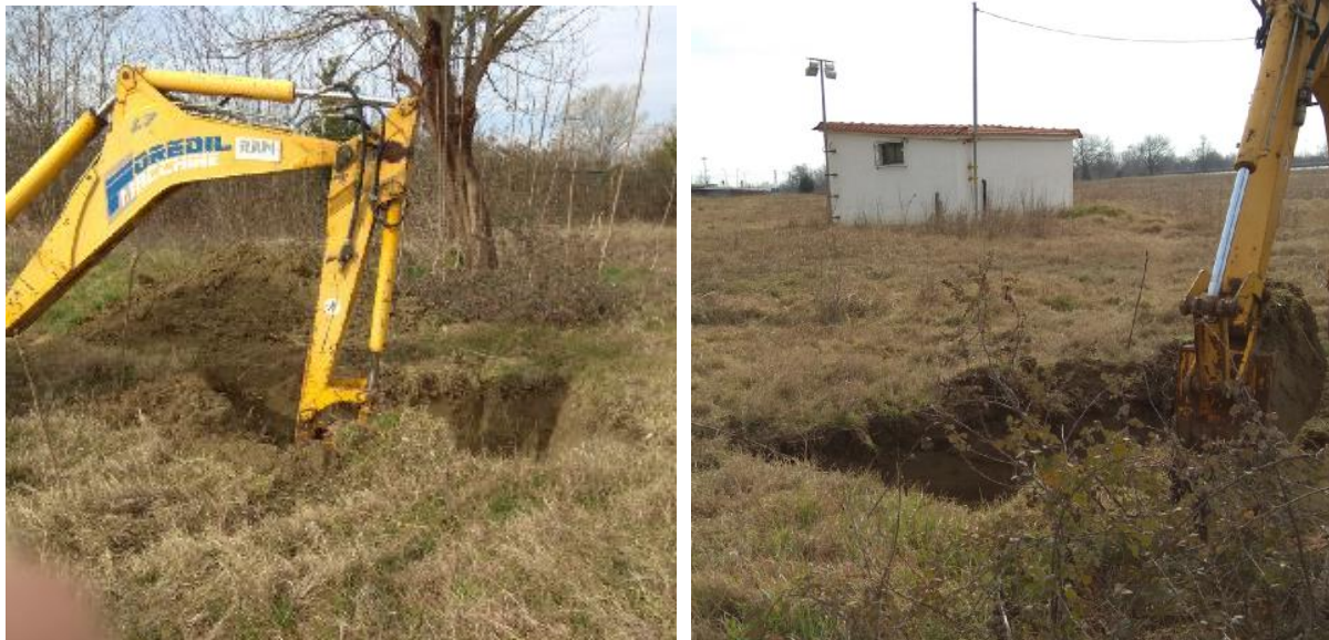
Figure 35. Excavation to host the drilling material
