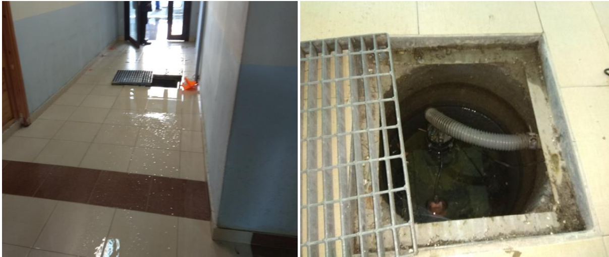
Figure 7. Water pump C1 installation at shallow depth inside the concrete casing.
