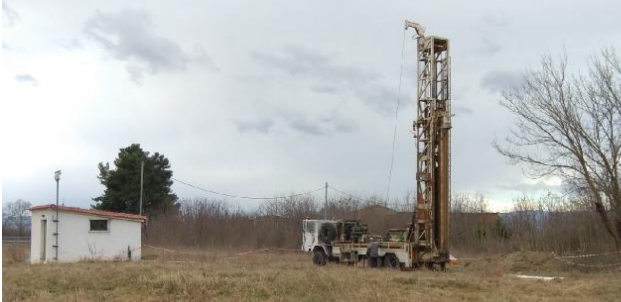
Figure 36. Installation of the drilling rig next to the excavation
