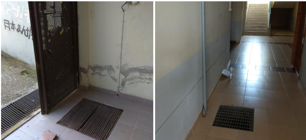
Figure 5. Water pumps B1 (Building B) and C1 (Building C) with protective grille covers
