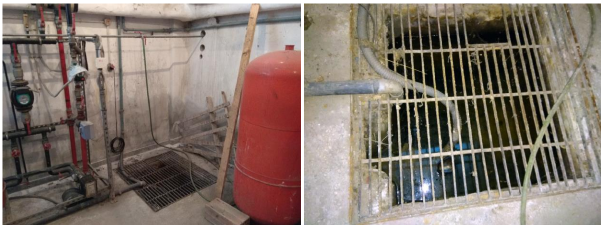
Figure 6. Water pump B2 installation at shallow depth inside the concrete casing
