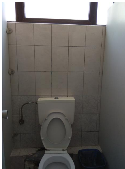
Figure 4. Typical toilet facility of Building B
