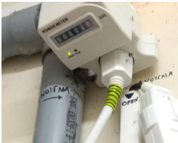
Figure 6. Power consumption measurements of existing water pumps in Building C (Pump C1 on the left and Pump C2 on the right, photo taken on 22/07/2019).
