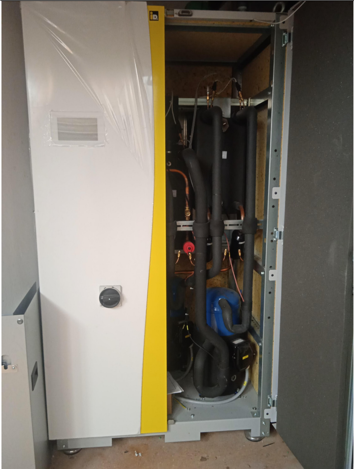
Figure 9. The inside of a heat pump
