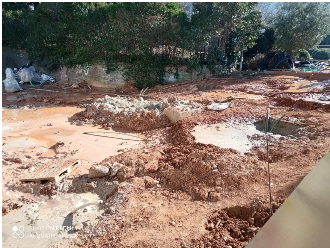
Figure 28. Filling the boreholes with grout
