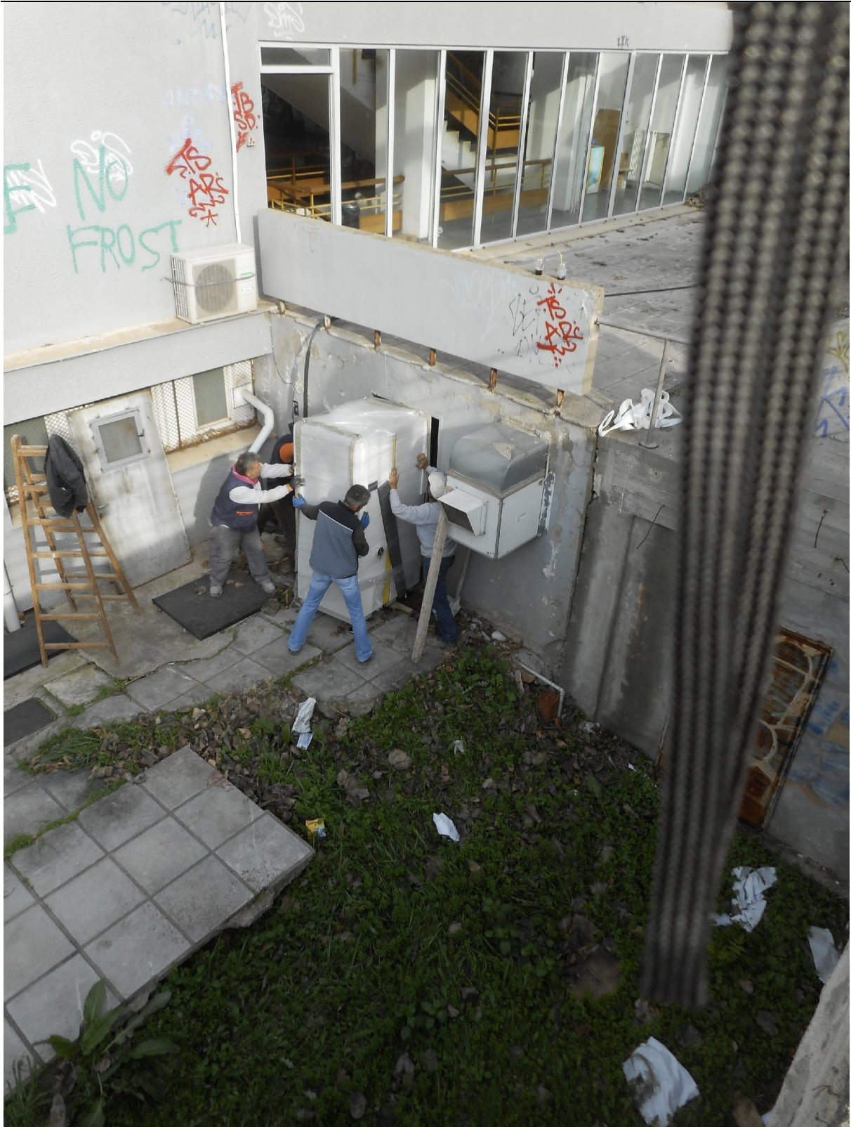
Figure 21. Bringing the heat pump inside the building
