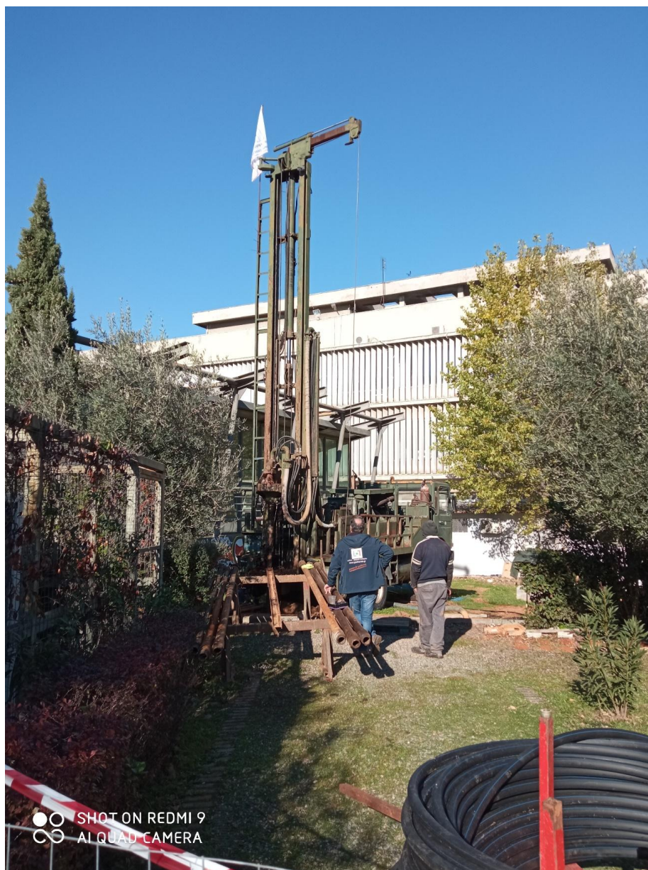
Figure 24. Borehole drilling equipment in situ
