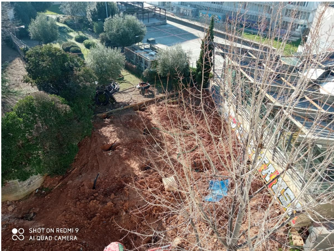
Figure 26. Geo-heat exchanger boreholes
