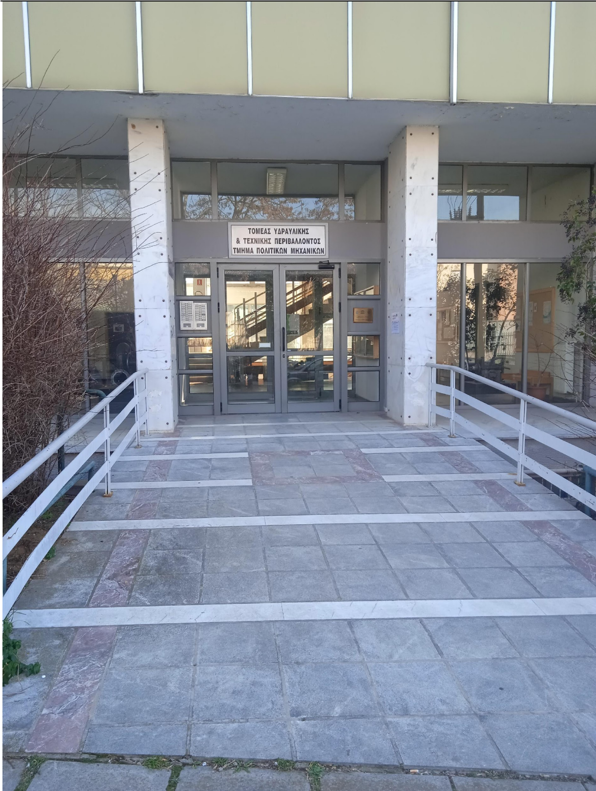
Figure 14. The entrance of the building of Hydraulics where the system was created
