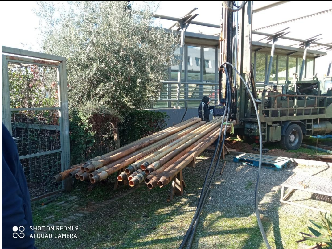
Figure 25. Tube installation in the boreholes
