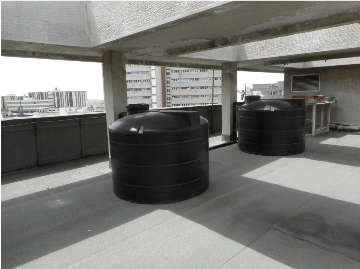
Figure 23. The location of the two water tanks at the roof of the building of Hydraulics
