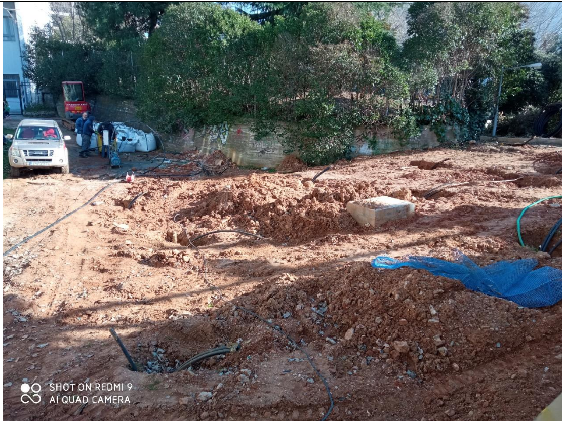
Figure 27. Geo-heat exchanger boreholes and the water well among them
