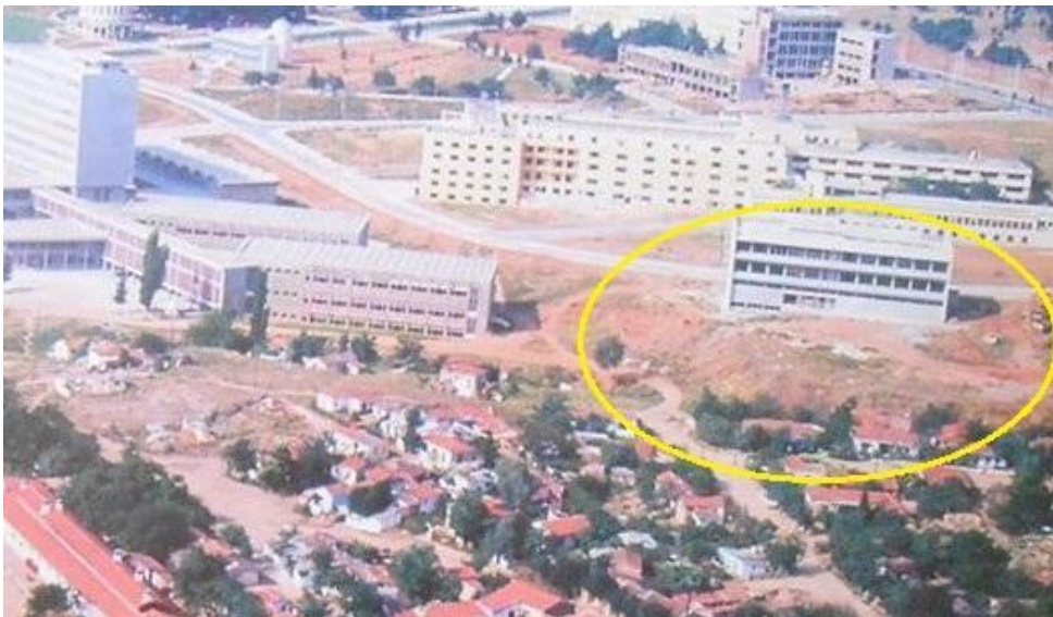
Figure 12. The site after the construction of the building of Hydraulics
