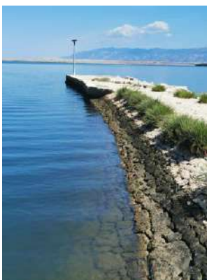
Figure 18. Inner side of the channel
