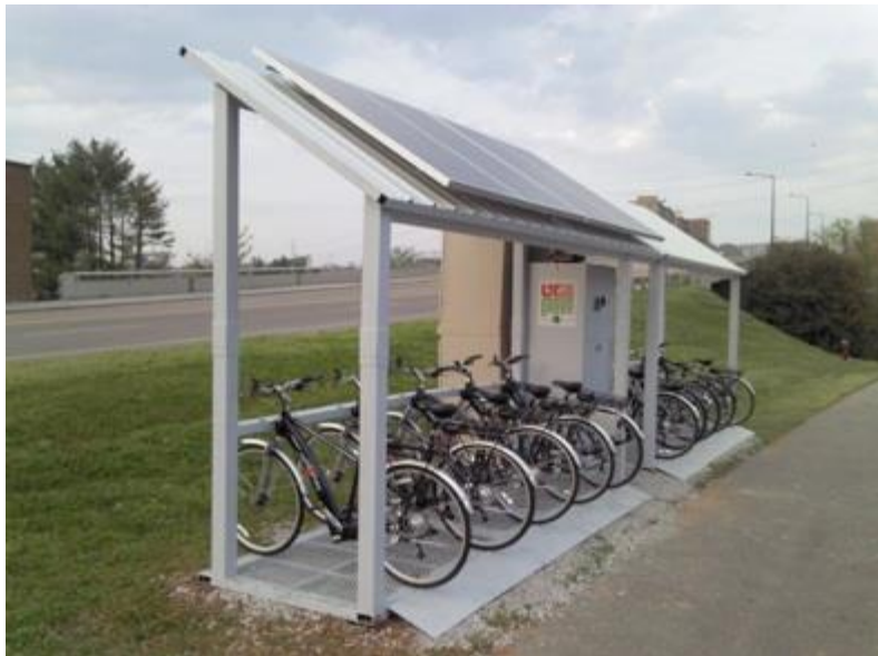
Figure 8. Solar powered station at the Knoxville campus (source: http://cycleushare.utk.edu/cycleushare/E-Bike_Sharing_at_UTK.html )
