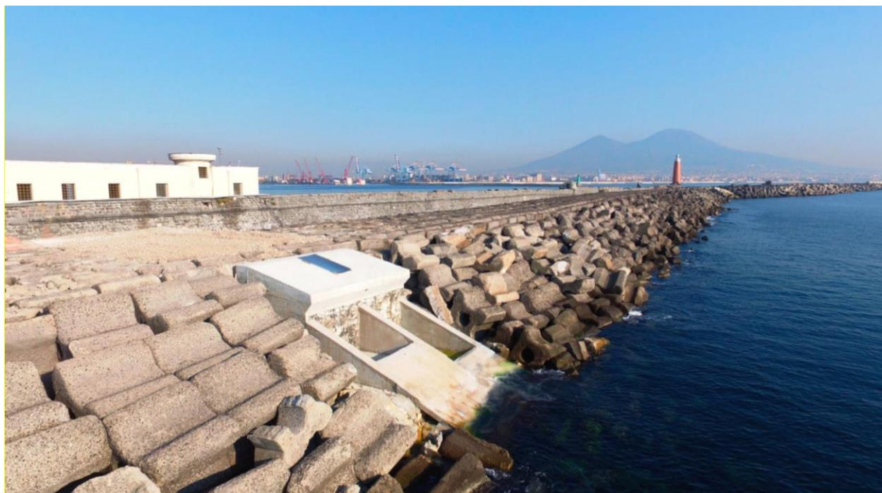
Figure 13. OBREC prototype in the port of Naples (source: Contestabile et al. 2016). The two reservoirs with their respective openings at different heights are clearly visible.
