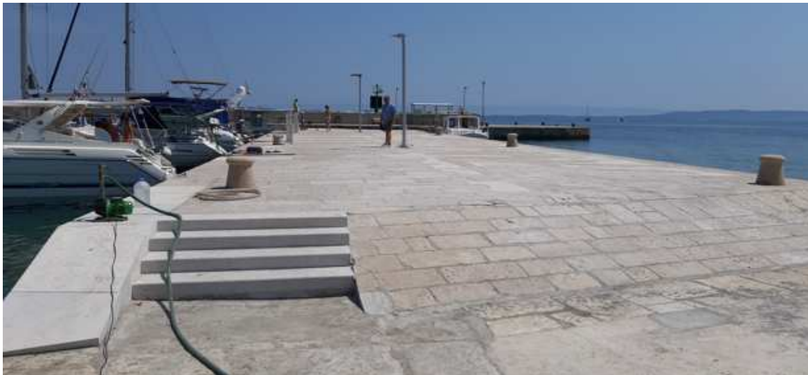
FIGURE 28. QUAY AT END OF WORKS.
