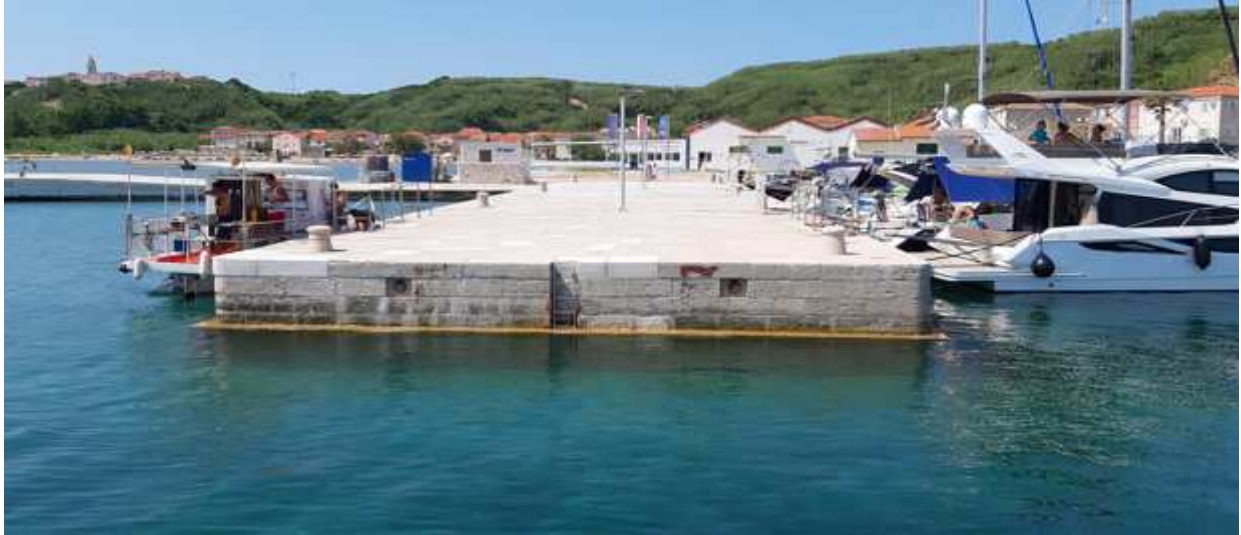
FIGURE 25. QUAY AT END OF WORK
