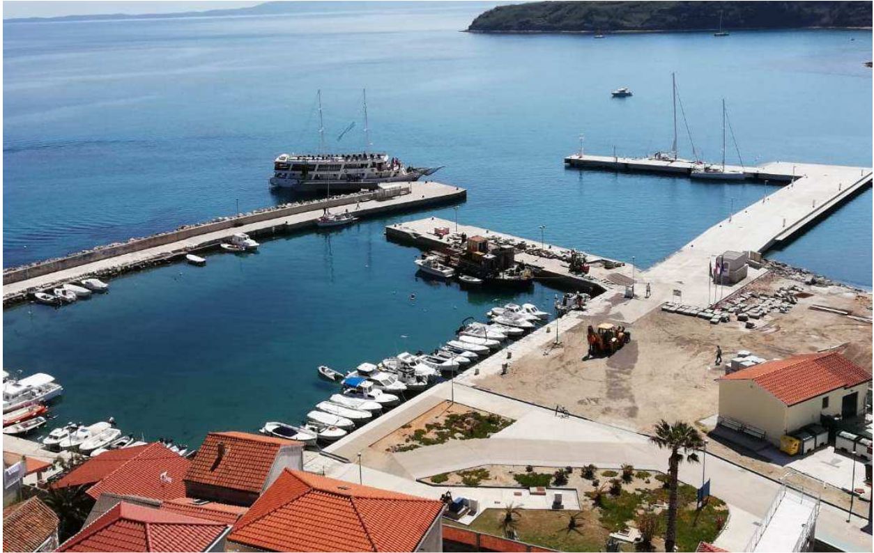
FIGURE 24. WORKS ON QUAY IN PORT OF SUSAK DURING THE MOSES PROJECT
