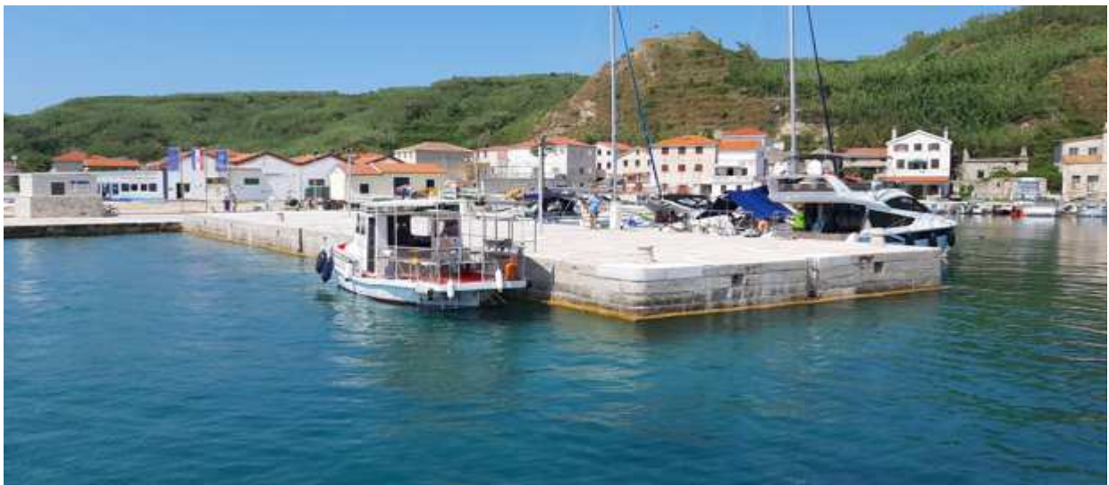
FIGURE 26. QUAY AT END OF WORK
