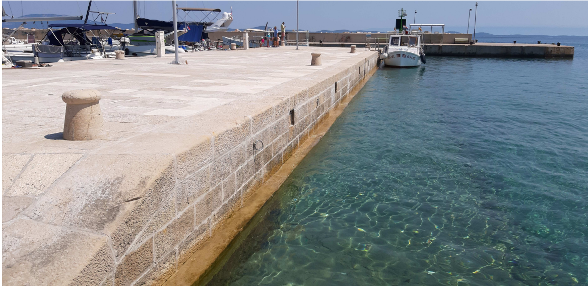
FIGURE 27. QUAY AT END OF WORKS.
