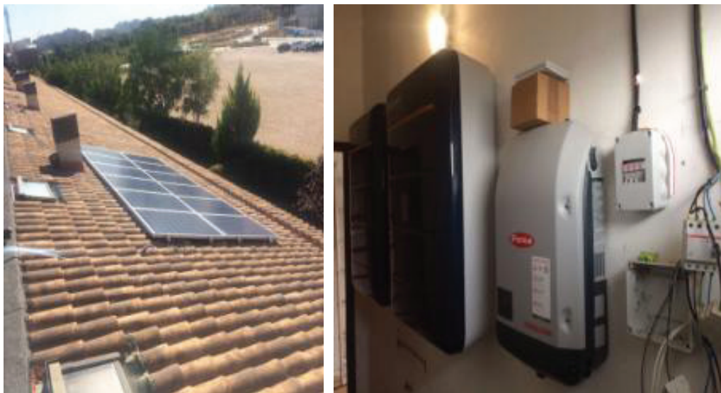
Figure 18 - Storage system of the second Spanish pilot (residential building)
