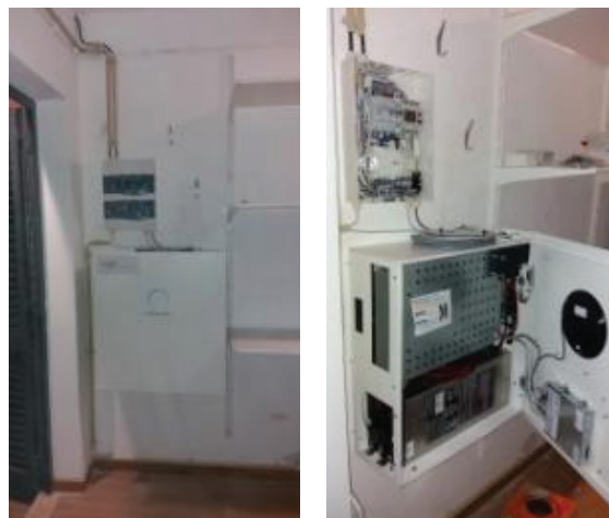
Figure 13 - Storage system of the third Portuguese pilot (residential building)
