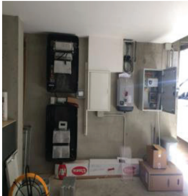
Figure 21 - Storage system of the fifth Spanish pilot (residential building)
