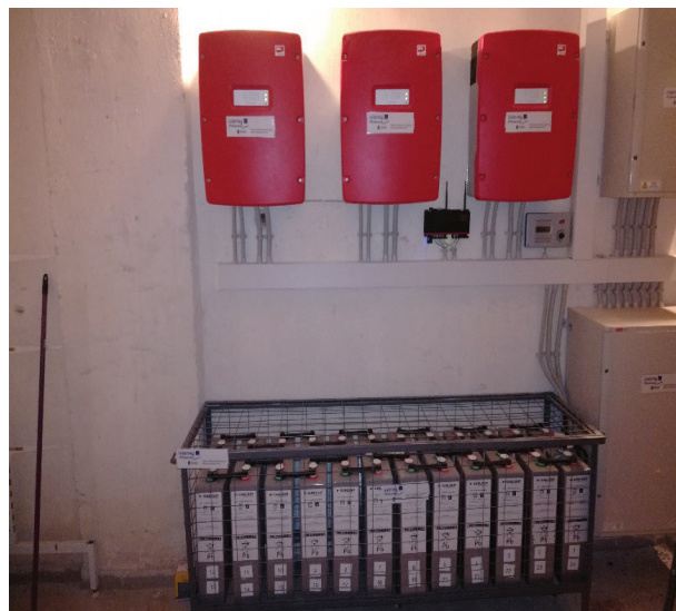
Figure 6 - Storage system of the first Greek pilot (public building)
