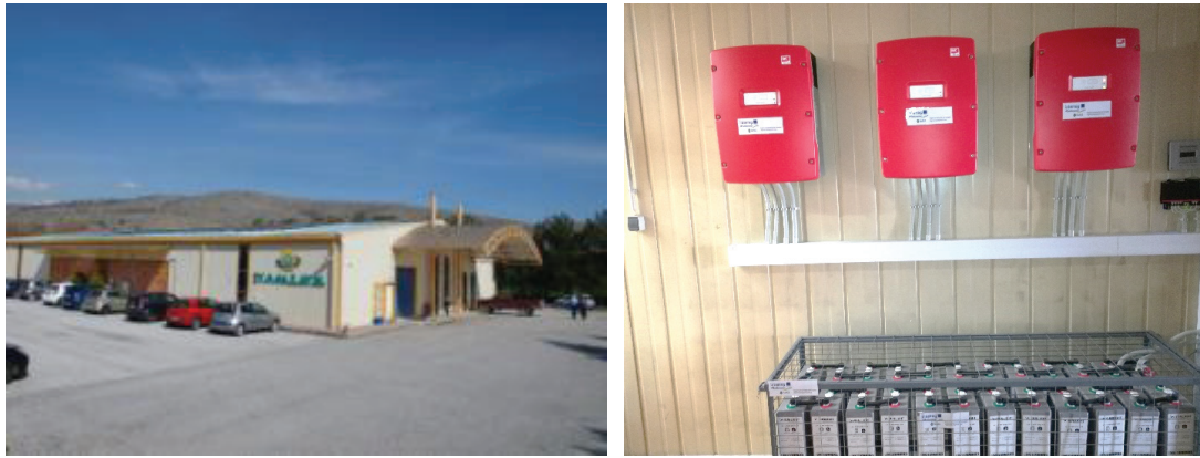
Figure 10 - Storage system of the fifth Greek pilot (commercial – office building)
