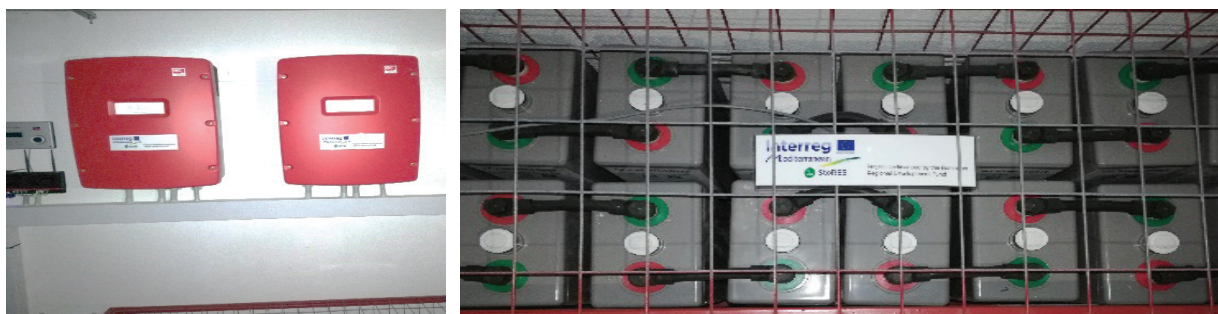
Figure 7 - Storage system of the second Greek pilot (public building)
