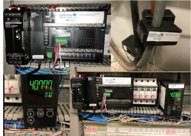
Figure 7 – Measuring system established for continuous monitoring of microgrid pilot in Slovenia
