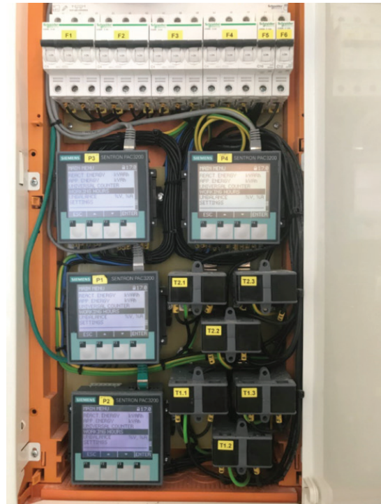
Figure 10 - Installed Siemens Power Meter in the Preko pilot microgrid
