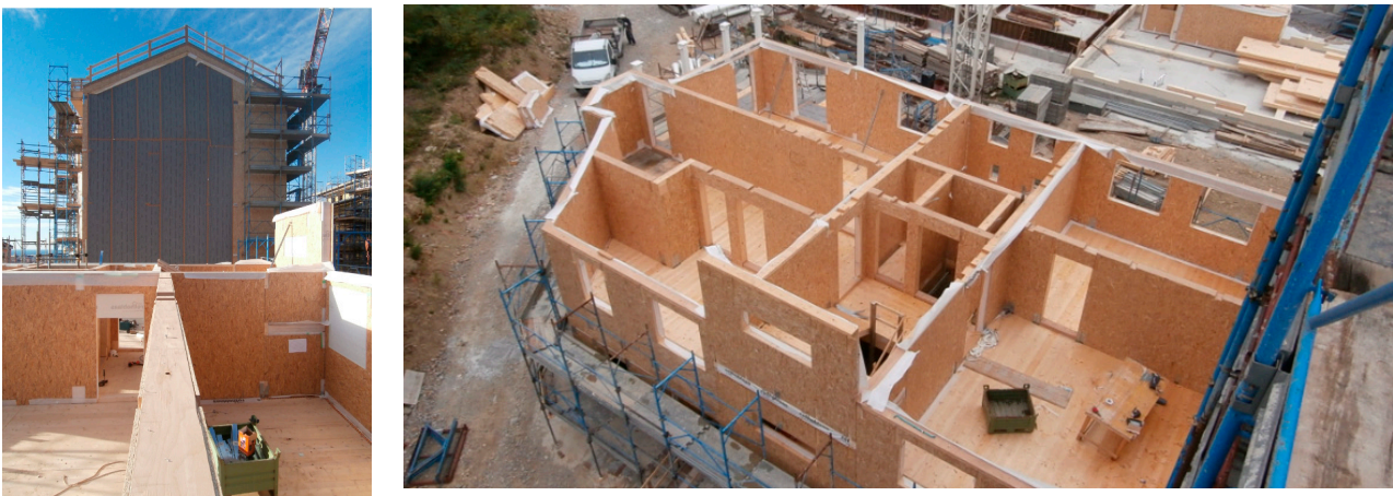
Figure 1. Realization of the test-building.
