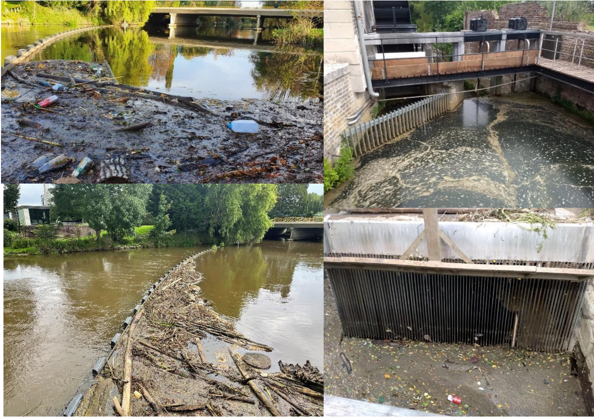
Figure 7 Left: Floating barriers Roer. Right: Duckweed/litter fences Geul (Grote Molen, & Rothermolen)
