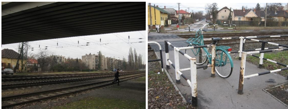
Figure 37: Left – Lack of crossings results in people crossing the railtracks at dangerous places Right – Even the crossings should be developed to make them suitable for bikes
