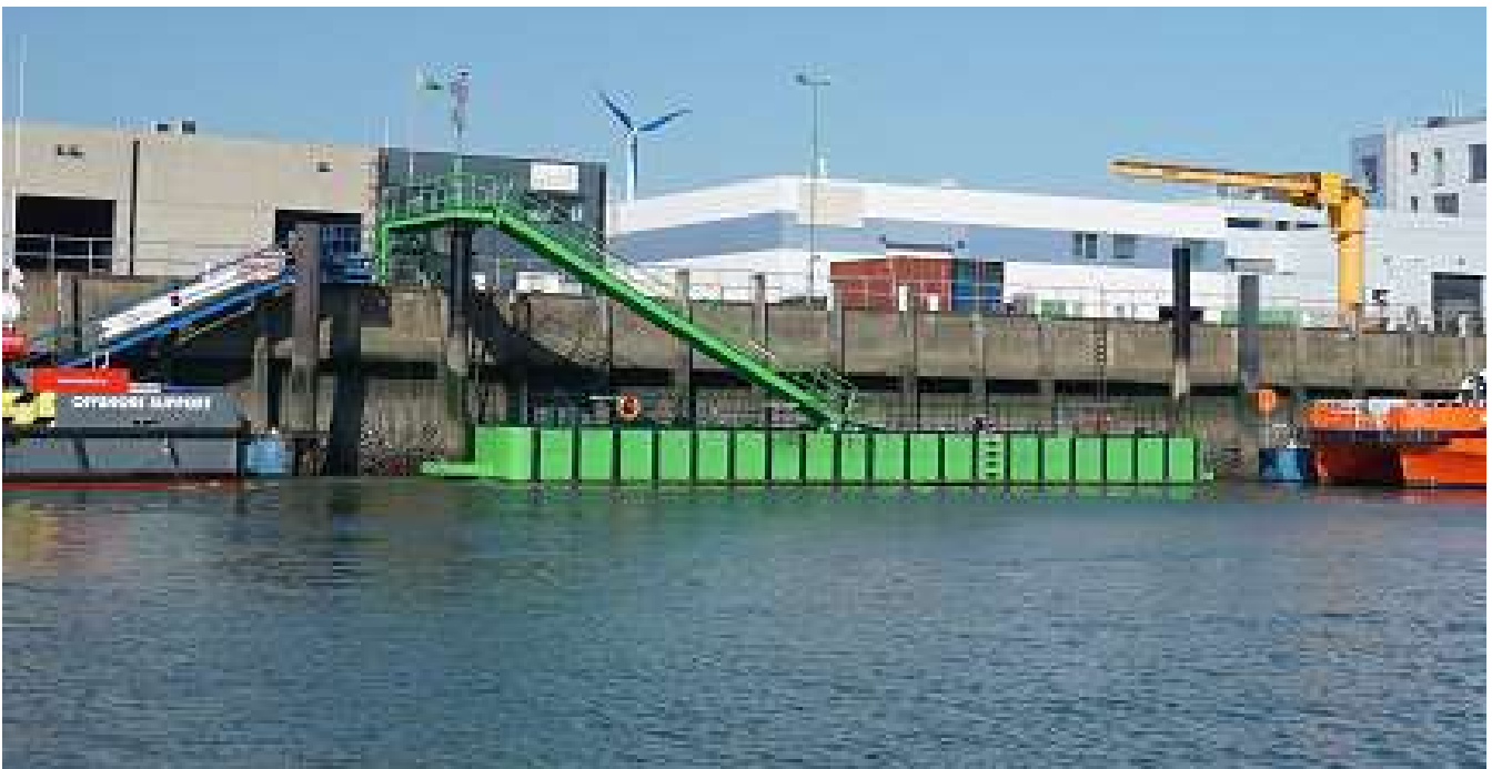
Figure 6.1 Smart LED-pontoon in the harbour of Oostende
