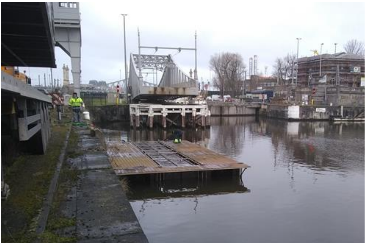
Once in the water the pontoon is moored. 2 Springs + fore and aft mooring rope.
