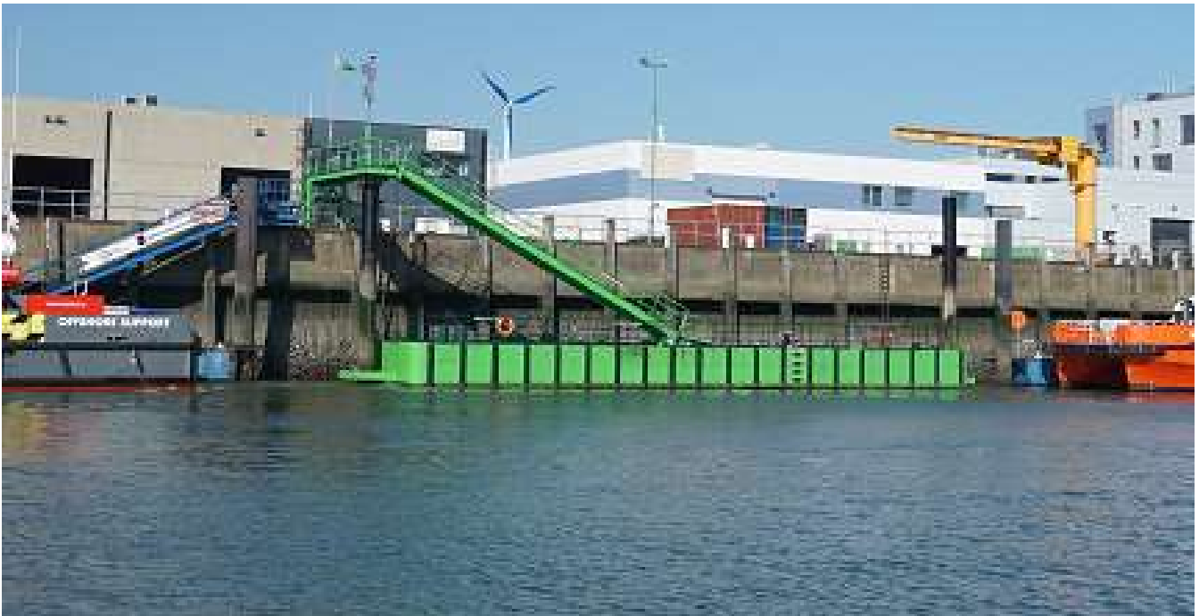
Figure 6.1 Smart LED-pontoon in the harbour of Oostende
