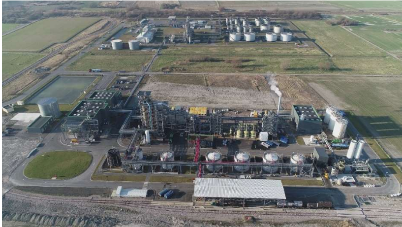
Figure 1 Aerial picture with in front the IndaChlor site and at the back Ryssen, with the direct steam connection between both sites visible.
