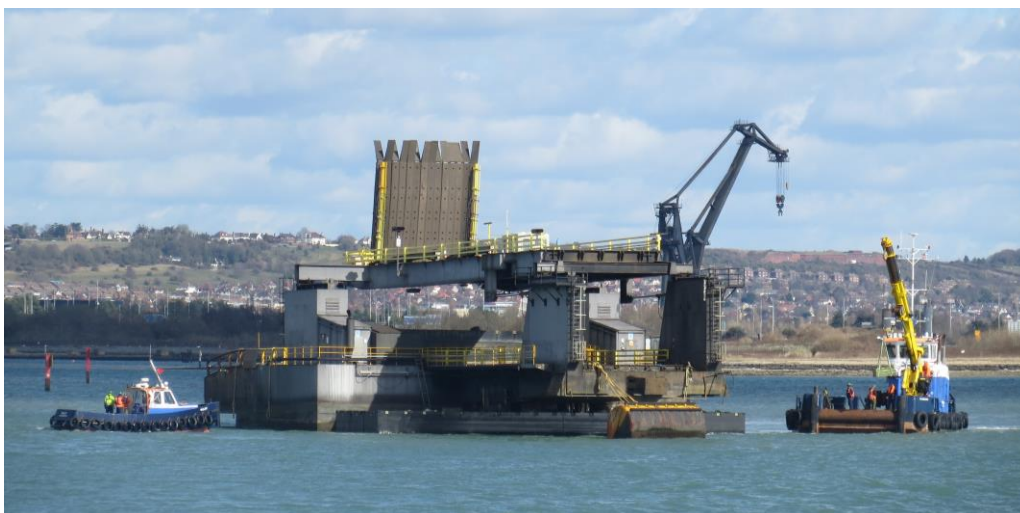
Photograph showing Old Linkspan at moorings following successful removal
