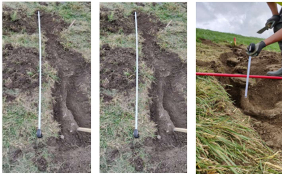
Figure 16: Excavated burrow structure after grouting.
