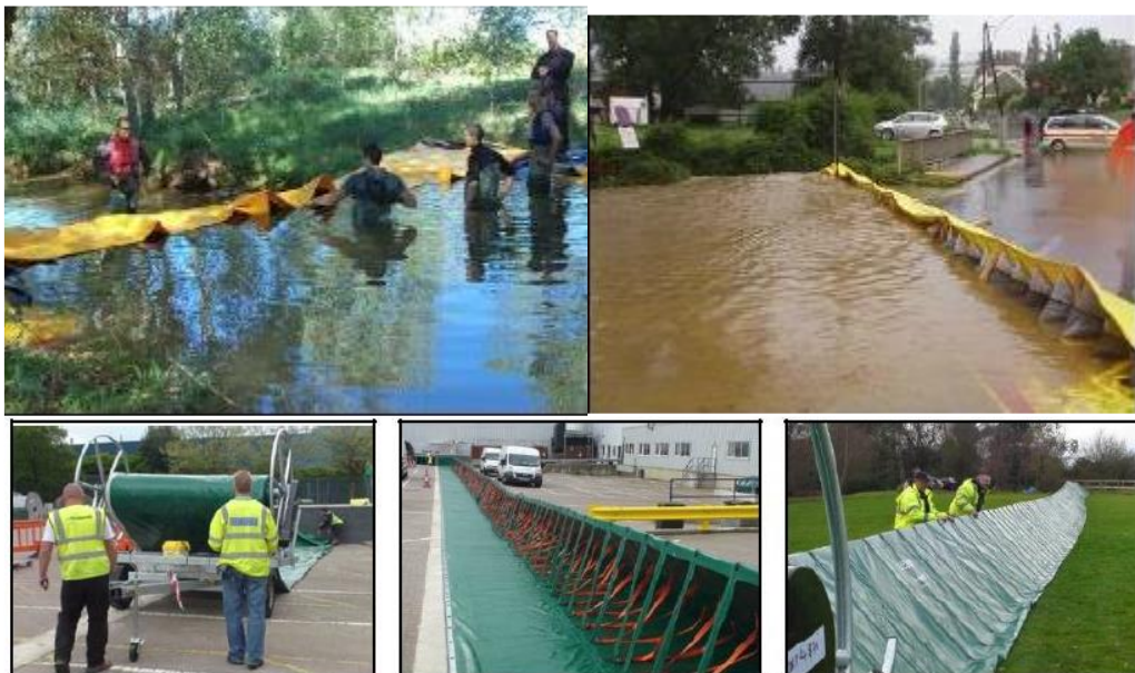
Fig. structures souples (Alteau, Watergate, Rapidam)
