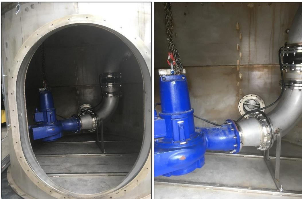
Figure 29: Amarex pump placed inside the tank
