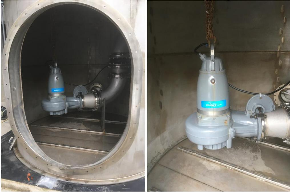
Figure 32: Flygt pump placed inside the tank
