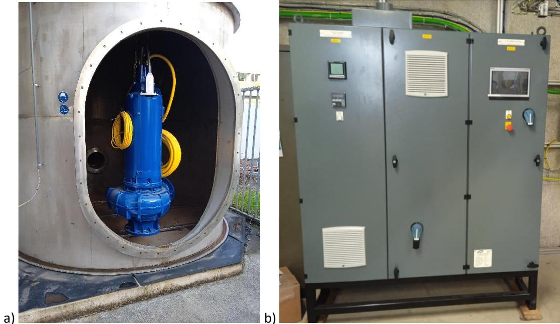
Figure 2.2: (a) Hidrostal pump placed inside the tank and (b) associated VFD
