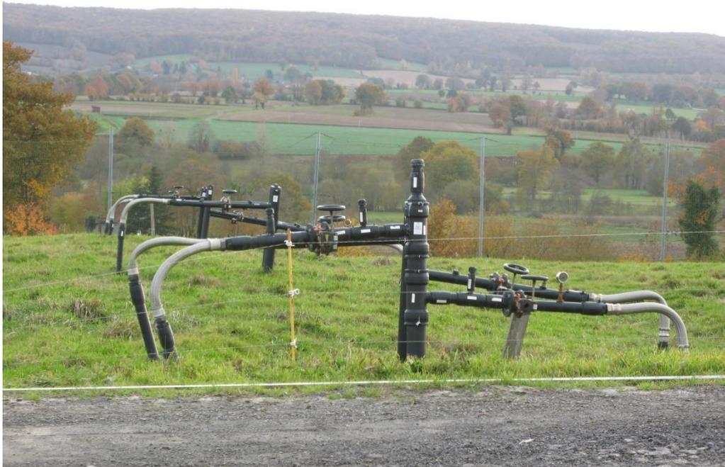
*Figure 3: Gas extraction and leachate recirculation system present on the landfill.*
