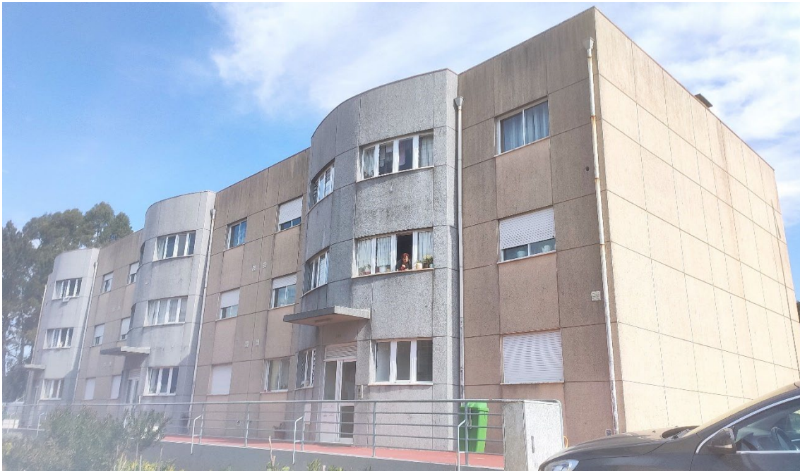
Figure 9: Studied social housing neighborhood before renovation.
