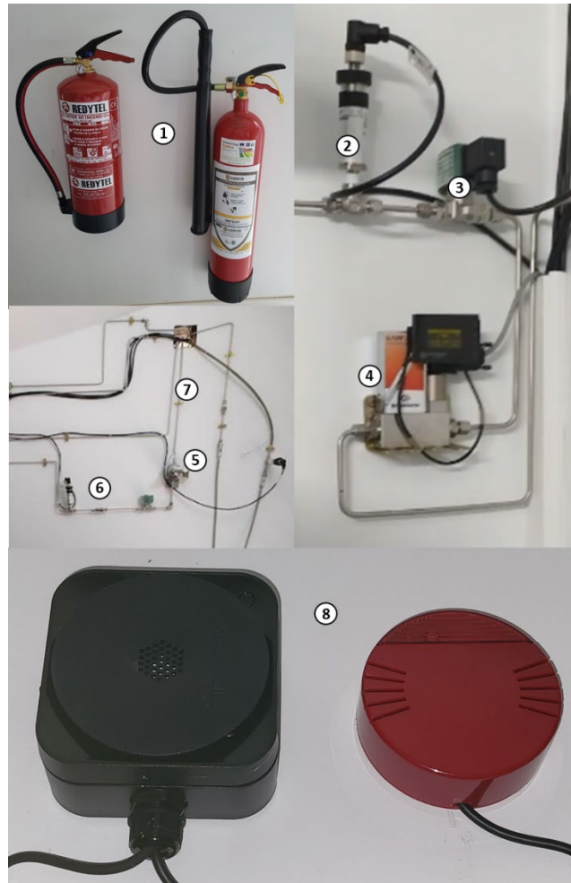
Figure 30: Fire extinguishers (1), pressure transducer (2), electrovalve (3), mass flow controller (4), pressure regulator (5), check valve (6), stainless steel piping (7) hydrogen detector and alarm (8).
