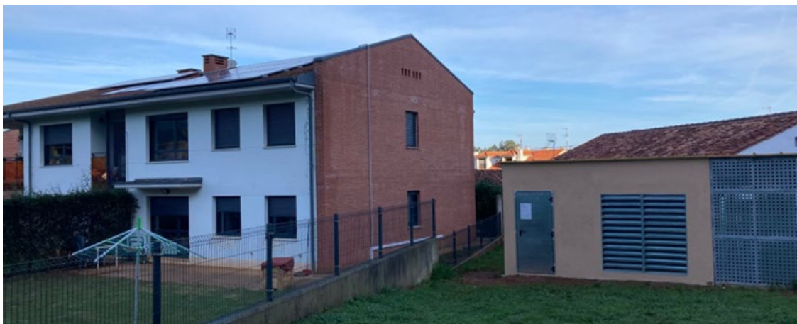
Figure 27: Housing and installation hut with pilot plant.
