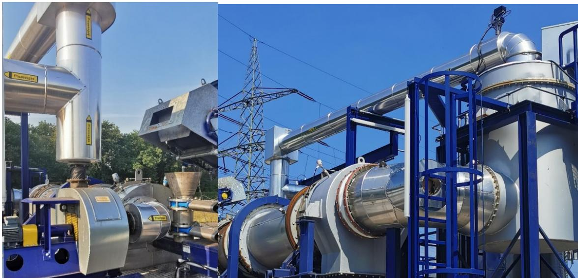
Figure 3.2.10 a and b: Gas split (flue/exhaust gas) and one of the two incineration chambers (Pictures: Emschergenossenschaft/L. Pamuk)
