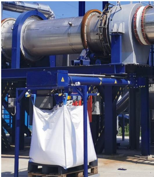
**Figure 3.2.9: SSA discharge at the EuPhoRe®-plant (Picture: Emschergenossenschaft/L. Pamuk)**
