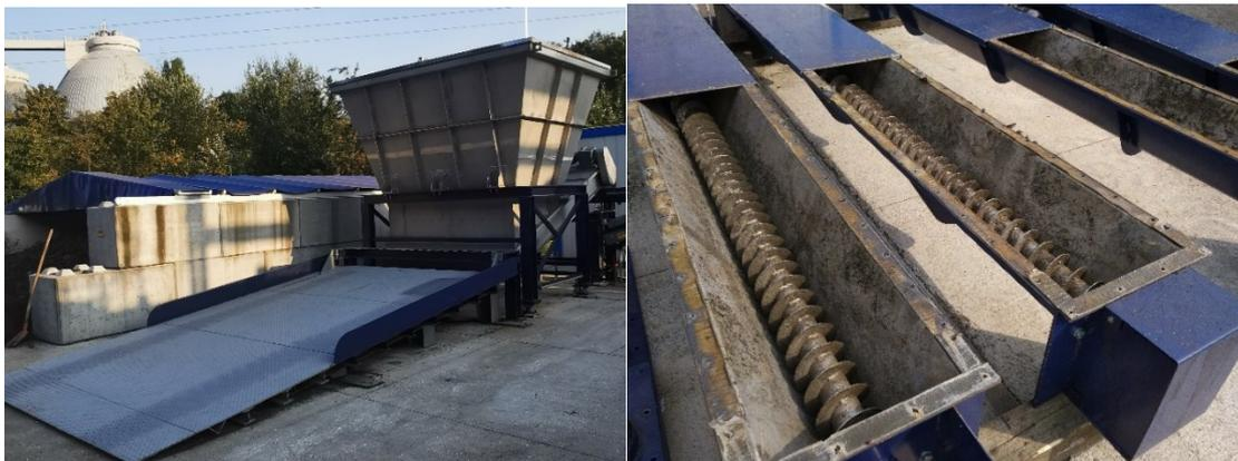
Figure 3.2.3 a and b: Sludge hopper and screws (Pictures: Emschergenossenschaft/L. Pamuk)
