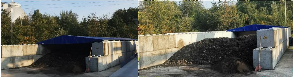
Figure 3.2.2 a and b: Sludge storage (Pictures: Emschergenossenschaft/L. Pamuk)
