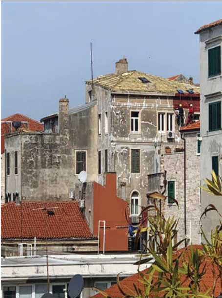
Facades before renovation
