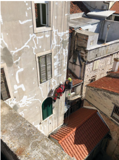
Facades before renovation
