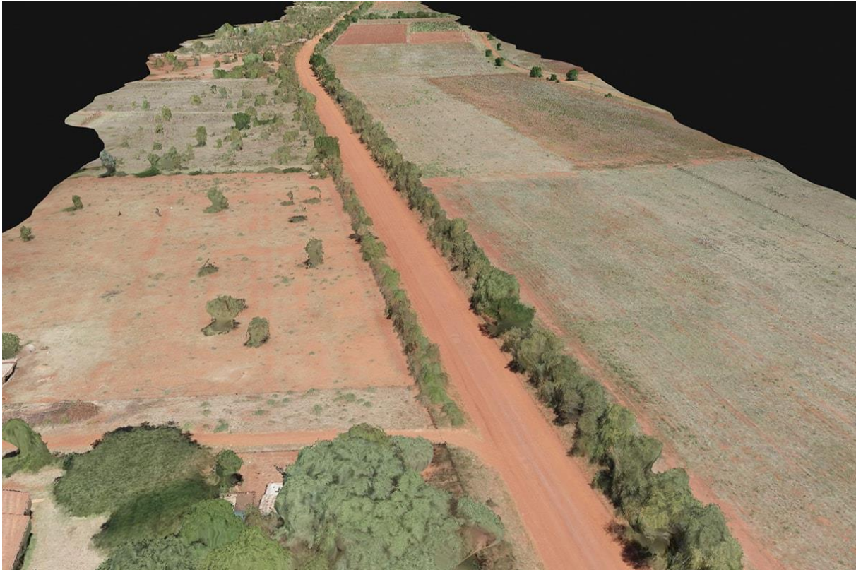
Fig.6 Survey of African road before construction planning (Image: By Wintgra, https://wingtra.com )
