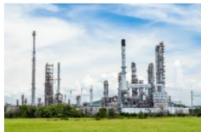
"Strengthening the administrative capacities of
