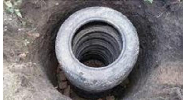
Figure 5. A DIY cesspool made of tyres.
