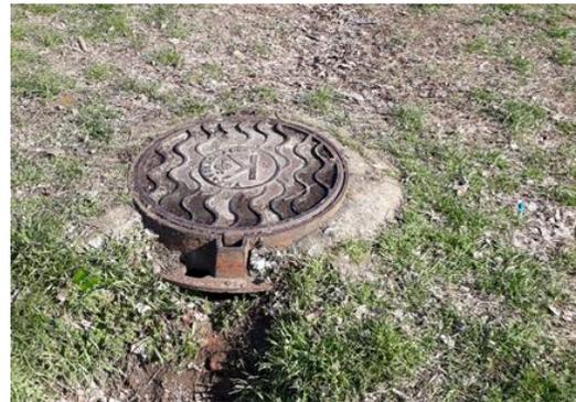
Figure 6. A manhole with a local sewerage system for greywater of a school in a rural area. The greywater pipe ends in a ravine, which can be transported to the river by the stormwaters.
