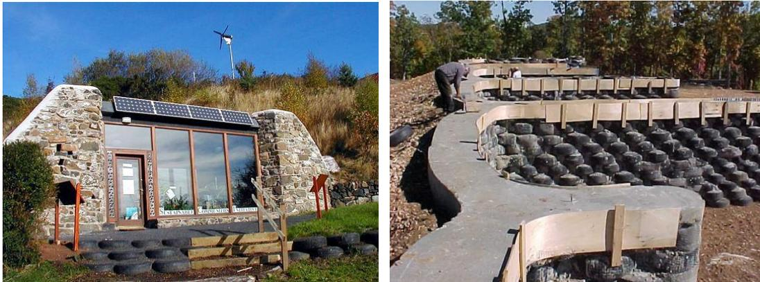
Figure 46. Re-use of old tyres in construction. Source: homedit.com
