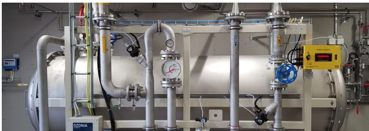
Figure 86 | Ozone generator tank at Nykvarn WWTP
