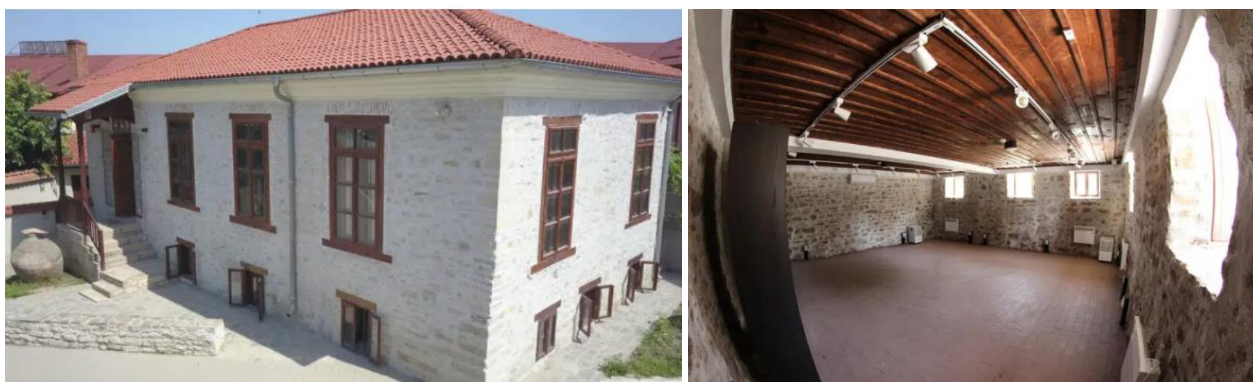
Fig 4 – Panaghia House, Babadag, Tulcea County , refurbished and modernized as a museum through ROP 2014-2020, Priority Axis 5, Investment priority 5.1: “Preservation, protection, promotion and development of the natural and cultural heritage.
