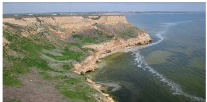
Image 11: Abrasion-landslide type of slope (Rybakivka village, 2020)
