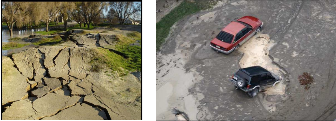
Figure 4: “Waves” of liquefied soil (left) and area severely liquefied (right). Photos from New Zealand Christchurch earthquake (M6.3, 21-2-2011) source: http://www.nzherald.co.nz .
