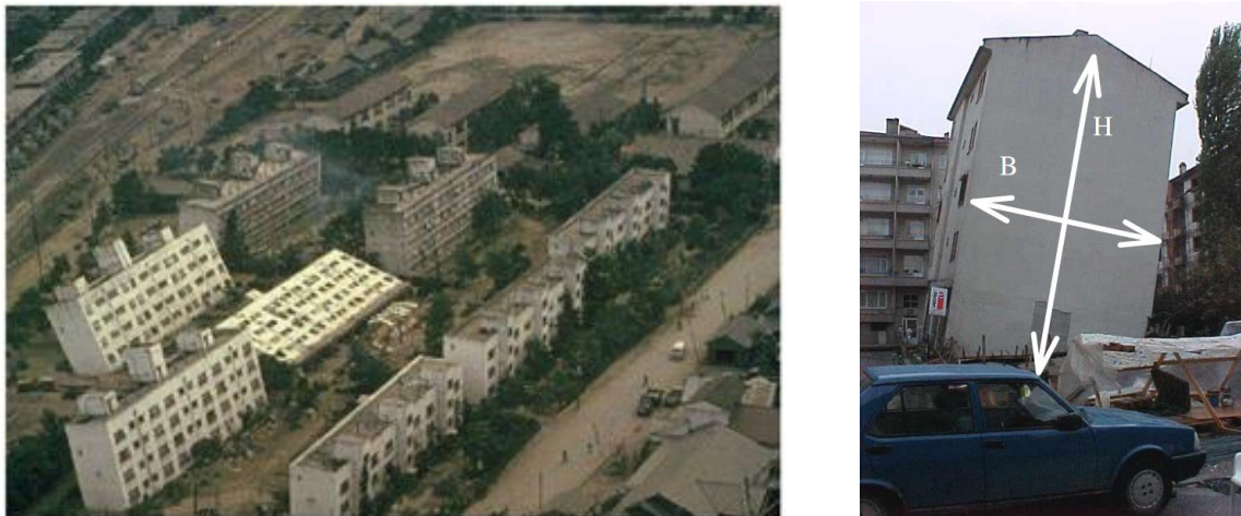
Figure 5: (left) Collapse of buildings due to soil liquefaction during the 1964 Niigata, Japan earthquake (photo: Joseph Penzien), (right) Vertical displacement with significant tilt of the building in Adapazari Türkiye, 17-8-1999.
