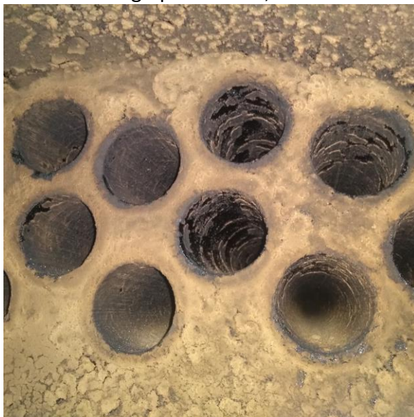
An example of tarring and sooting in heat exchangers due to poor quality fuel and inadequate cleaning
