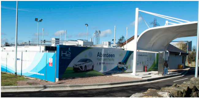
Figure 23: Aberdeen City Hydrogen Energy and Storage station (ACHES)
