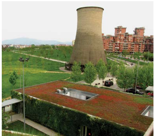
Photo 7: Examples of green infrastructure - green roof
