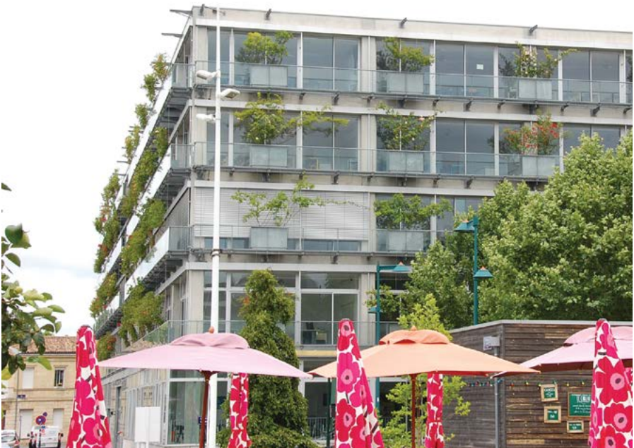
Photo 4: Examples of the green infrastructure on the buildings
