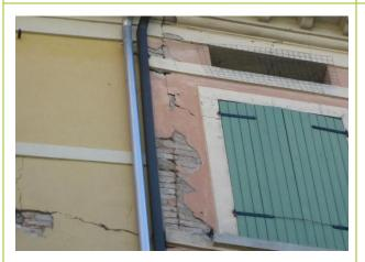
Lacking of connections between the walls
