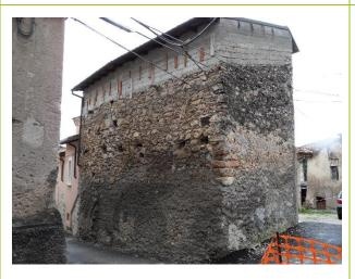
Raising of a stone masonry building with concrete blocks, probably for the renovation of the roof
