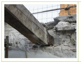
Poor connection between roof and walls
