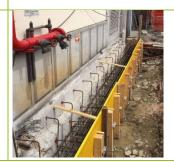
Continuous reinforced concrete foundations (strip footings)
