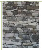
Dry tuff masonry (assimilated to rubble stone masonry not well organized and without connection between the two wall surfaces for its behaviour).
