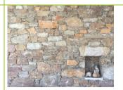
Rubble masonry with regular sized stones, well organized but without connection between the two external surfaces, with the presence of edges, bundles and / or courses in square stone or solid bricks.
