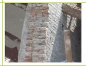
Rubble masonry with bricks on the surfaces and in the internal core, well organized but without connection between the two external surfaces realized with bricks and the internal core
