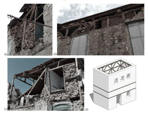
Figure 24 – Localized out-of-plane collapse of external unreinforced leaf and schematic sketch of timber-frame masonry (Vlachakis, 2020)
