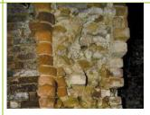
Rubble masonry with bricks, well organized but without connection between the two external surfaces realized with bricks, with the presence of edges, bundles and / or courses in square stone or solid bricks.
