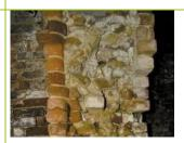
Rubble masonry with bricks, well organized, but without connection between the two external surfaces, with the presence of edges, bundles and / or courses in square stone or solid bricks.
