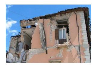
Figure 26 - Representation of the "beam effect" of the RC tie beam on masonry walls
