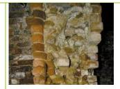
Rubble masonry with bricks, well organized but without connection between the two external surfaces realized with bricks, with the presence of edges, bundles and / or courses in square stone or solid bricks.
