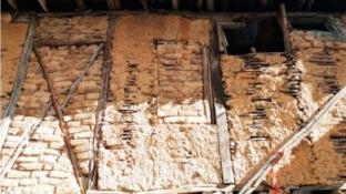
Figure 21 – Veroia: Timber-framed traditional house; construction details of the exterior wall (Mousourakis, 2020)
