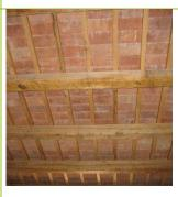
Single or double timber floors (beams and joists) with brick tiles
