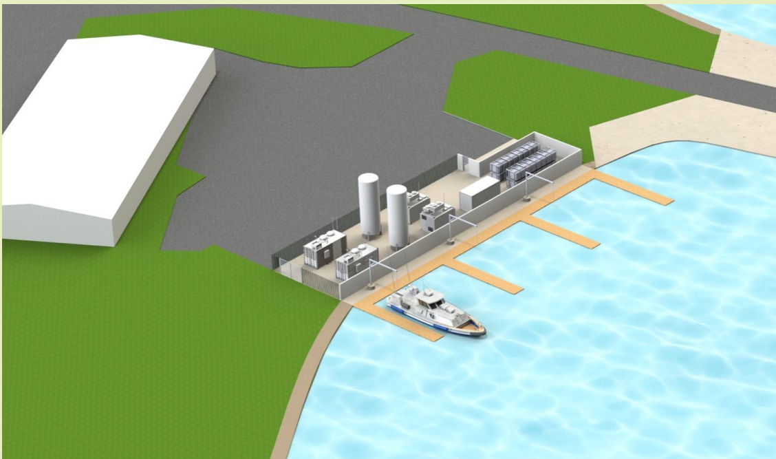
Figure 15. Concept render of a 2MW hydrogen bunkering system
