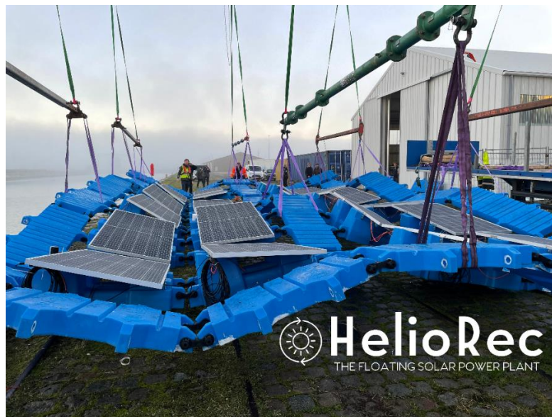
Figure 3: Lifting test in Oostende Port
