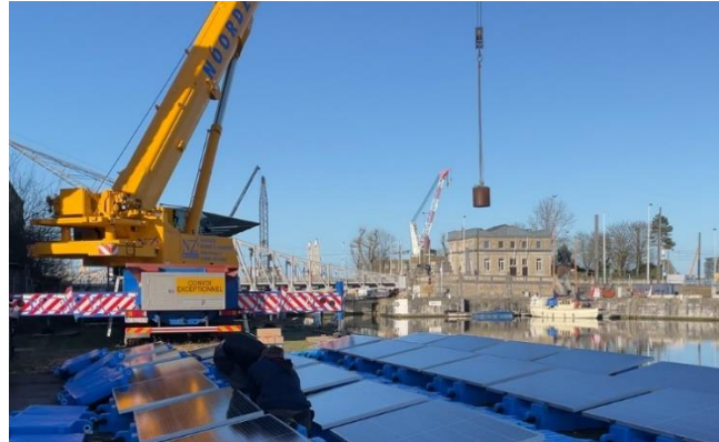
Figure 6: Anchor block positioning
