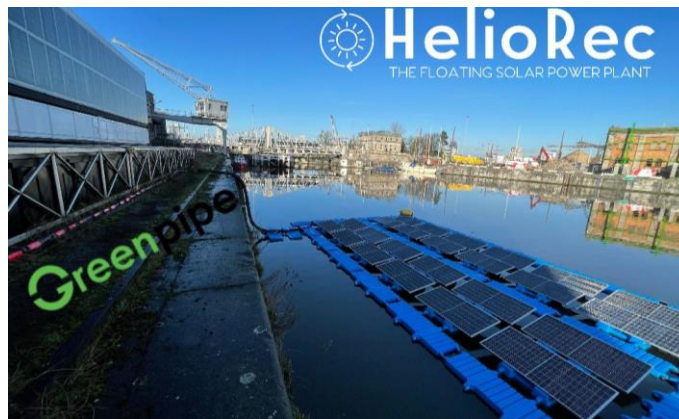
Figure 2: Floating solar power plant in Oostende port
