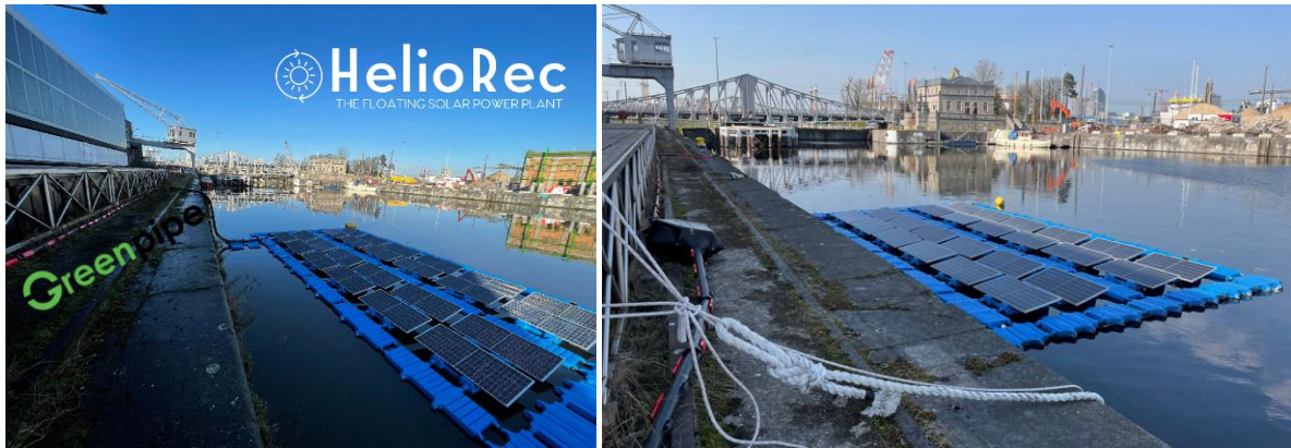
Figure 4: DC cable protected with Greenpipe’s divisible cable protection pipes.
