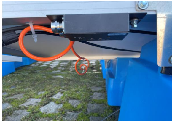
Figure 8: Accelerometer connected to solar panel
