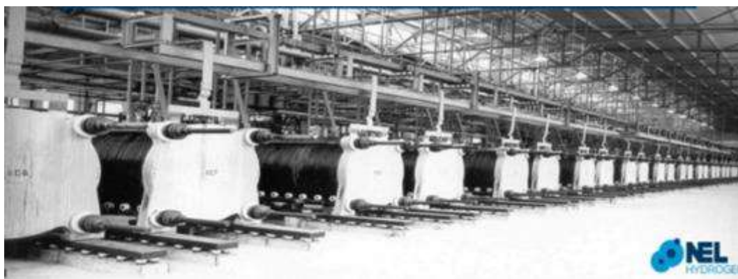
Figure 1 – A 135-MW alkaline electrolyser facility in Norway, operational from 1953 (NEL Hydrogen)
