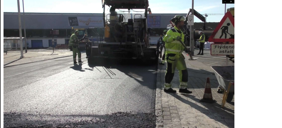
Figure 5: Roadwork at the Port of Skagen September 2020.
