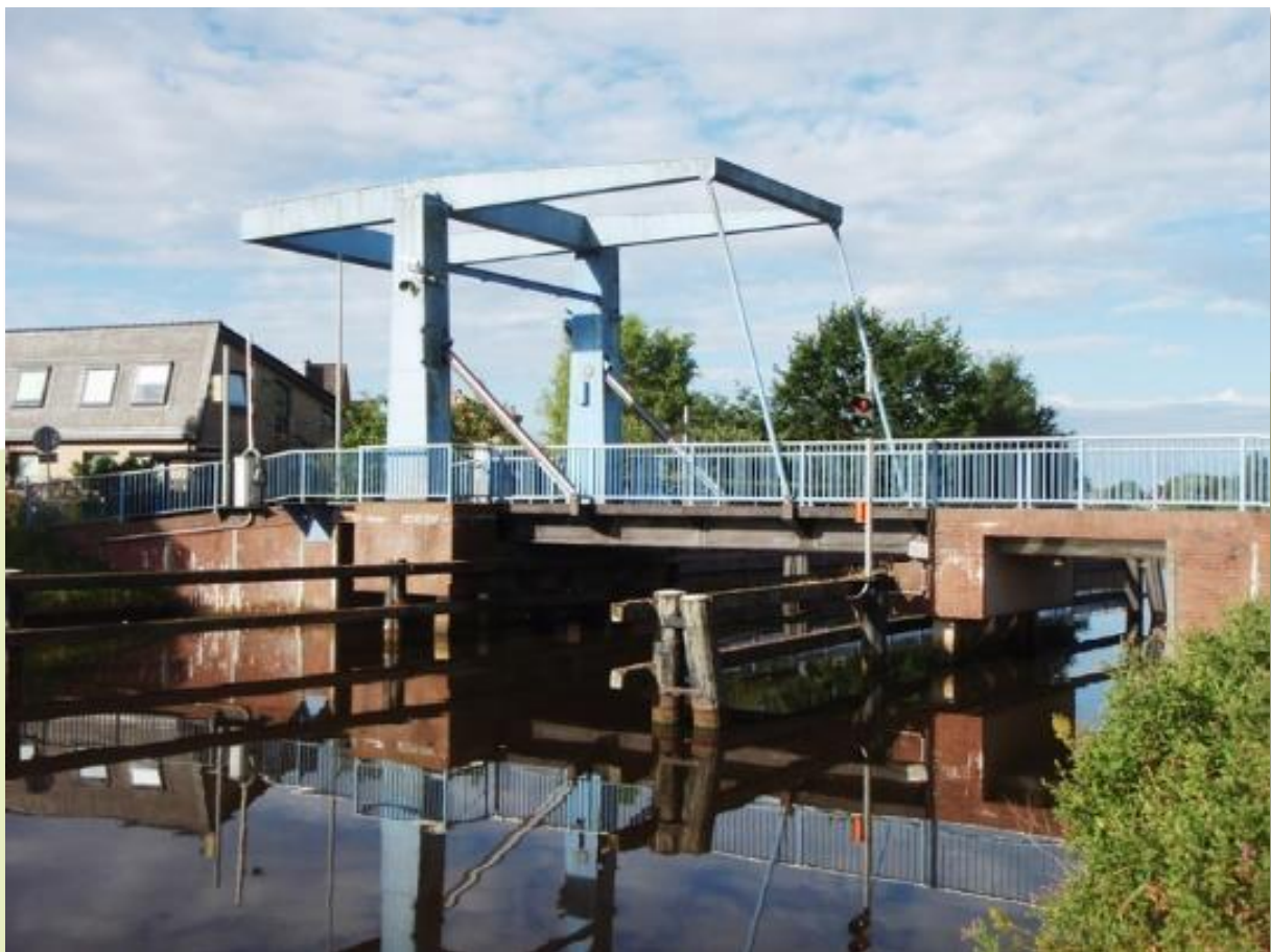
Figure 22. The bridge Wolthuser Brücke over the Ems-Jade-Kanal in Emden. Credits: NLWKN.
