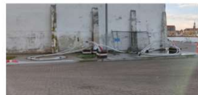
The area that is prepared for the transformer and inverter technology
