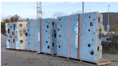
Connection points prepared for the boxes in the quay
