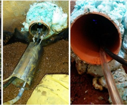
Figure 8 Suction strainer on crimp sleeve, Flowmeter and hereafter suction strainer during installation in the drainage pipe at the P filter inlet and Area Velocity Flowmeter.
