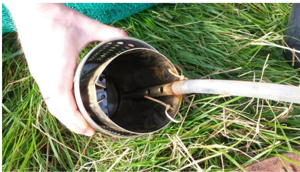
Figure 9 Suction strainer on crimp sleeve and in grid basket during installation at the outlet of the P filter.
