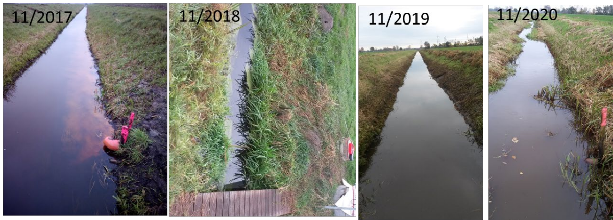
Figure 6 Different flow conditions in the Venner Bruchkanal in relation to the degree of clearance of the watercourse at the beginning of the drainage season in november from 2017 to 2020.
