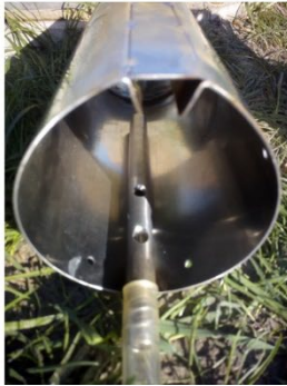
Figure 8 Suction strainer on crimp sleeve, Flowmeter and hereafter suction strainer during installation in the drainage pipe at the P filter inlet and Area Velocity Flowmeter.
