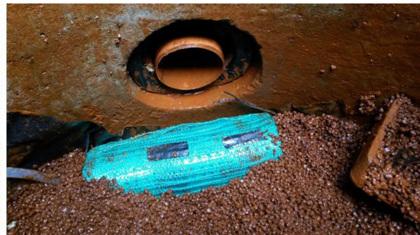
Figure 9 Suction strainer on crimp sleeve and in grid basket during installation at the outlet of the P filter.
