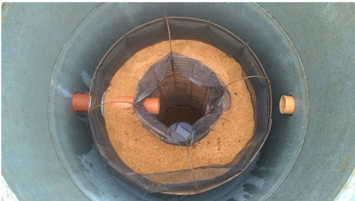
Figure 4 Reactive filter for dissolved P consisting of filter cage filled with Diapure™.
