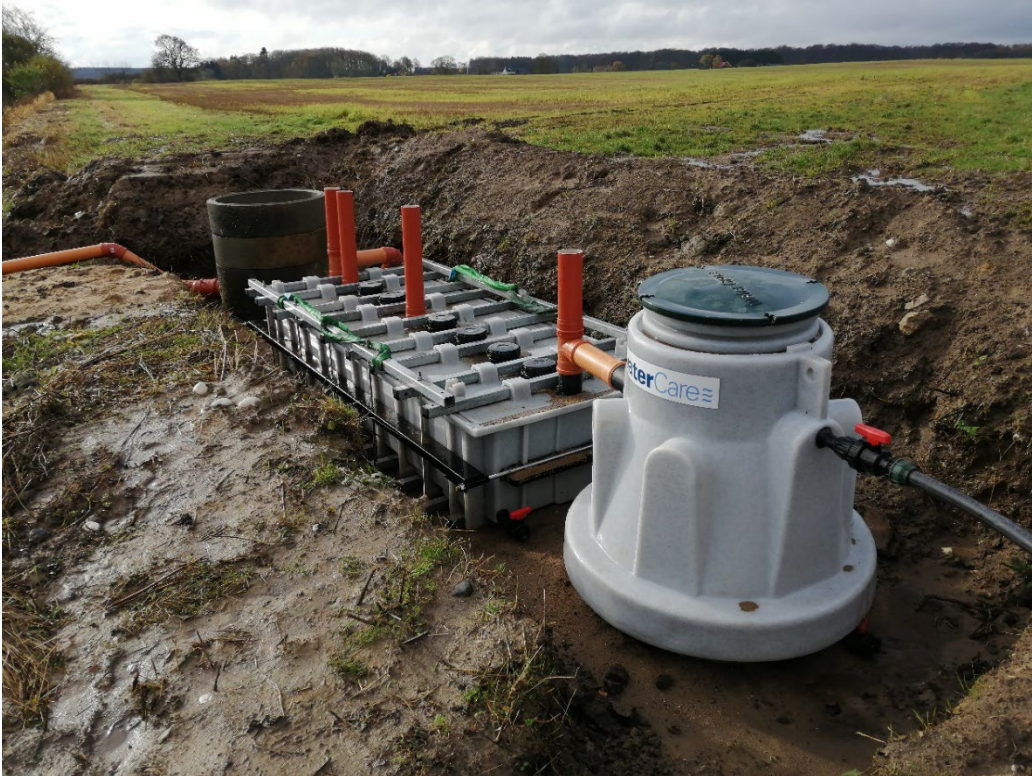
Figure 3 WaterCare™ prefilter for retaining sand and larger particles (right) and DPF sediment filter (left) during installation.
